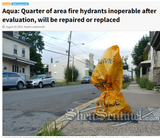
Photo 1. Inoperable fire hydrant bagged by Aqua until replaced. Shensentinel newspaper, August 10, 2023.
